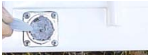
Figure 1 – Applying Silicon Dielectric Compound
